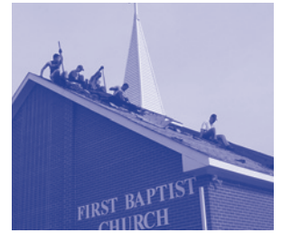
First Baptist Church in Wayland roof project
