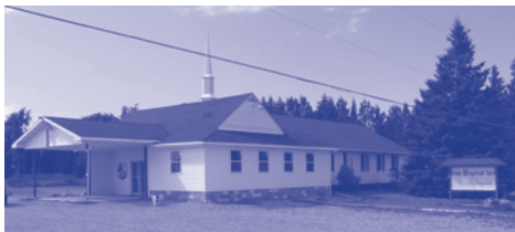
New renovated facilities of Brimley Baptist Church
